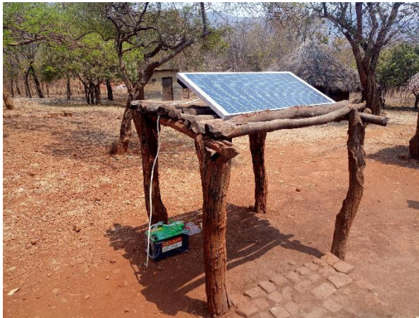
Off-grid power supply from a solar-battery system (left); The mobile-closed chamber system (right)
